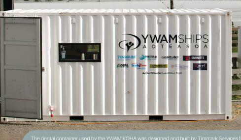
Whanganui. The self-contained unit houses dental equipment, an x-ray unit, an autoclave, fresh vater storage, gray water storage, a heat pump and a generator.
